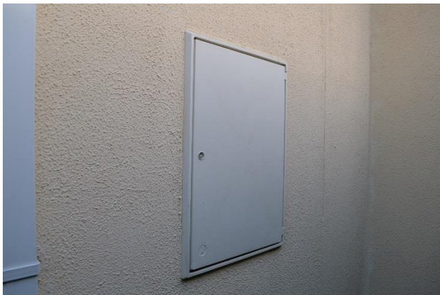
Typical Electricity Meter
